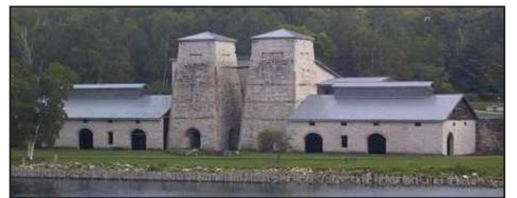
A BLAST FURNACE at the Fayette site is a modern-day survivor.
