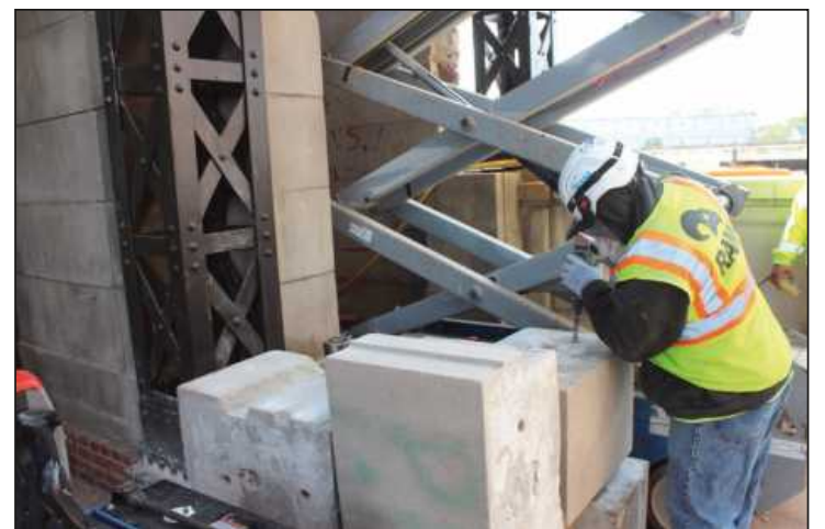
DRILLING A HOLE in a limestone block that will be re-set and re-mortared into the carriage house project at the Michigan Central Station in Detroit is Arthur Booker of Laborers Local 1191. He's employed by Ram Construction.
