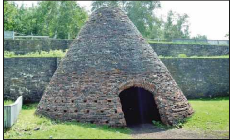
IT'S HARD TO BELIEVE this Medieval-looking structure was a kiln to make charcoal during the Industrial Revolution – but they used it at Fayette in the pig-iron making process from 1867-1891.
